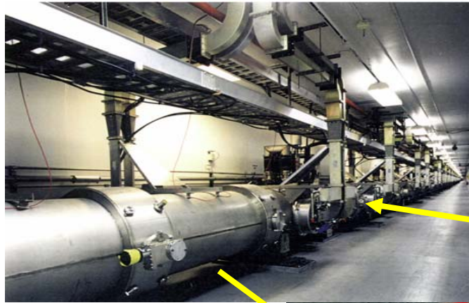
Cryomodules in the accelerator tunnel
