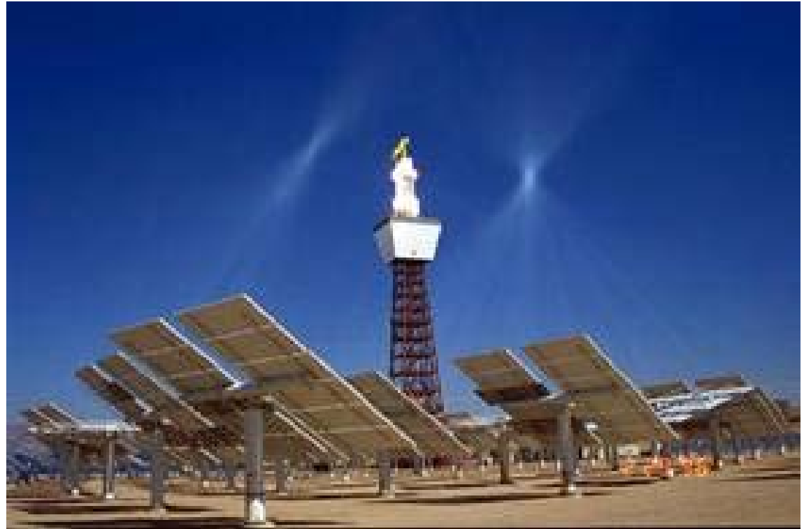
100 MW Solar Thermal Electric Project in South Africa
