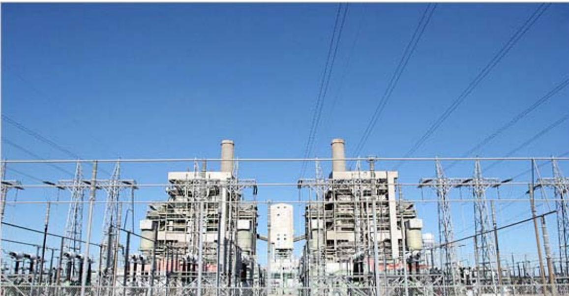
The two coal-burning units at TXU's Big Brown facility in Fairfield, Texas. (Misty Keasler for The New York Times)
