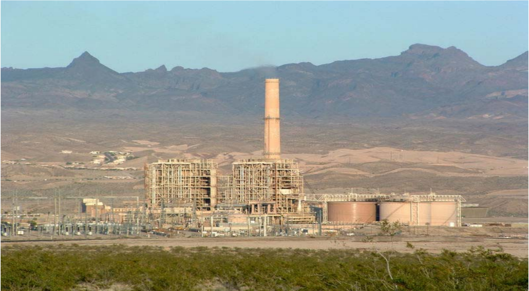
Mohave Generating Station, a 1,580 MW coal power plant near Laughlin, Nevada
