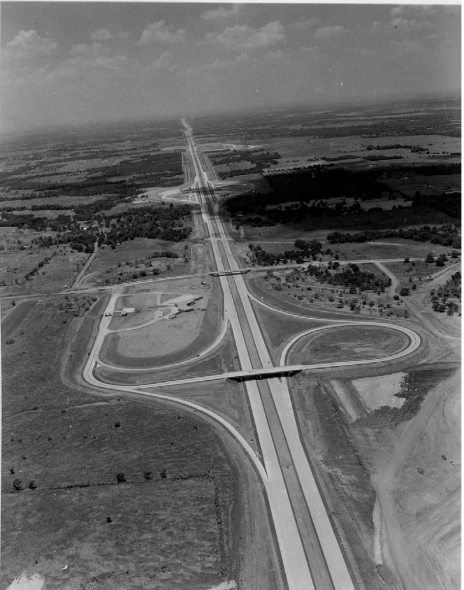
1936 Dallas-Ft. Worth Turnpike near Dallas
